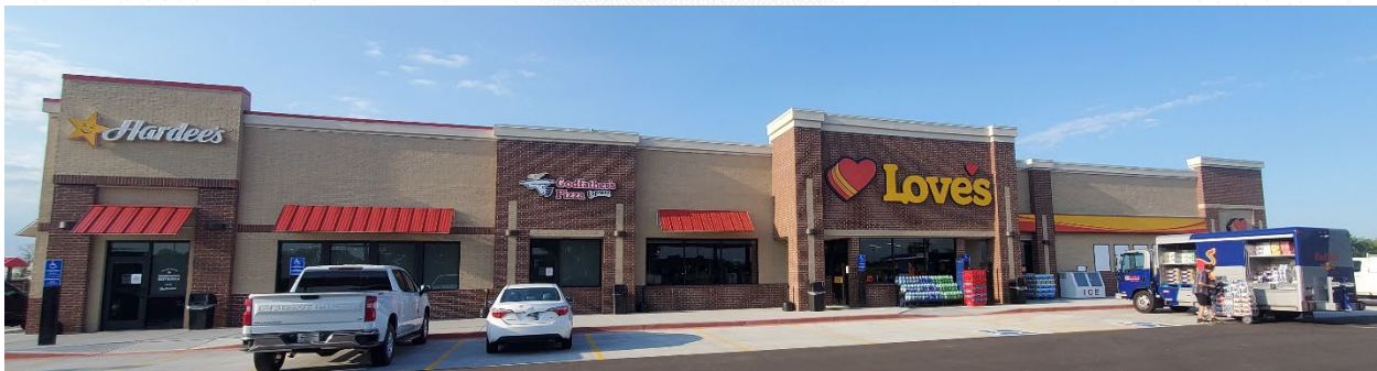
Front Entrance to Love's Travel Stop & Country Store. Address: 15402 Hornsby St. NE
