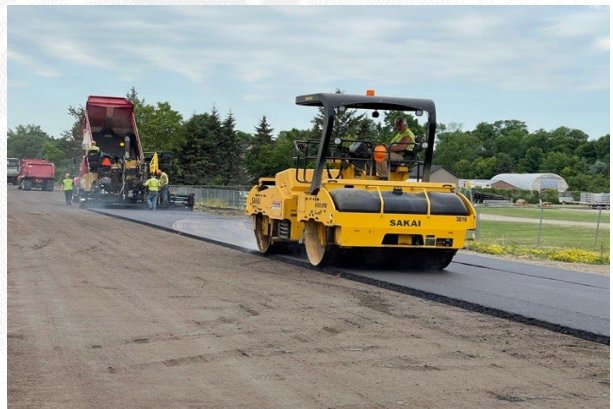
Paving of Hornsby Street in June of 2021
