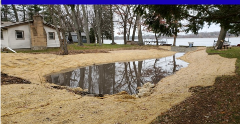
Stormwater pond rehabilitation—Martin Lake
