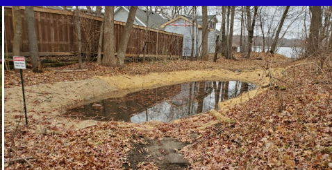
Stormwater pond rehabilitation—Martin Lake
